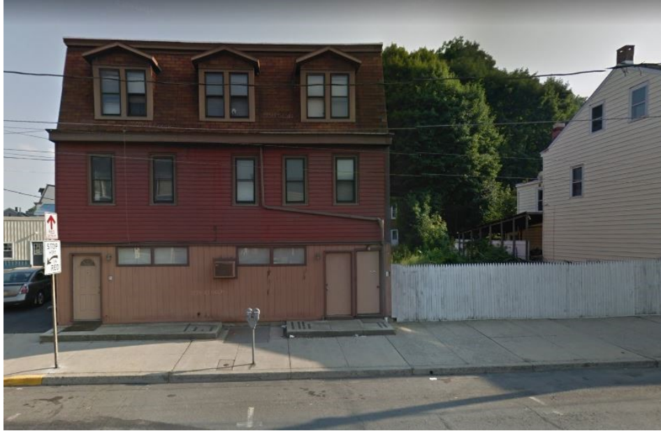
Minersville 11-13 Sunbury Street as it generally looks today.
