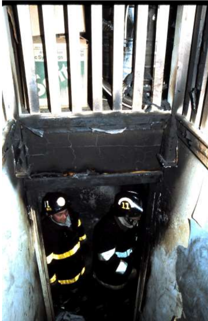
Veteran Engine 11 firefighter Dennis Fehr (left) and Lt. Mike Glore (right) in the 2 nd floor hallway in this view looking down from the attic stairs. Crews prevented the fire from extending into the attic area.
